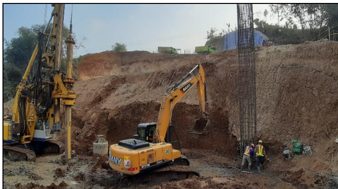
Bored piling works for a toll road in West Java, Indonesia
