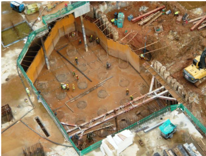
Bored piling works for a toll road in West Java, Indonesia
