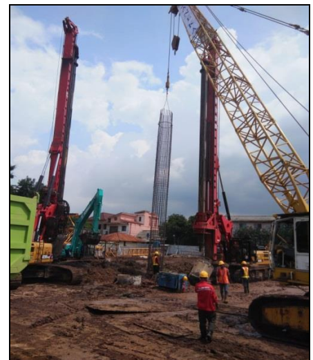
Bored piling works for a low cost apartment in Jakarta, Indonesia
