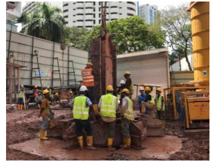
Installation of plunge-in column for an office tower in Kuala Lumpur
